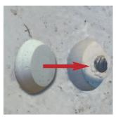
After removing the flange glue in the fine-grained concrete cone into the circular recess
